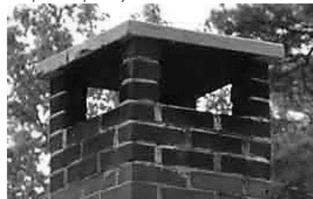
Concrete Cap Chimney Top
